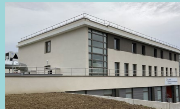
Extension of Saint-Omer private hospital, Blendecques (Pas-de-Calais) operated by Elsan – Completion: November 2023
