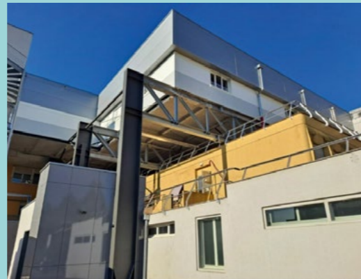
Extension of the operating suite at Les Cèdres private hospital in Brive-la-Gaillarde (Corrèze) operated by Elsan – Completion: June 2023
